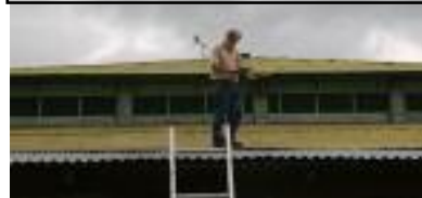
Joseph Moreno evaluating the building for panel placement.
